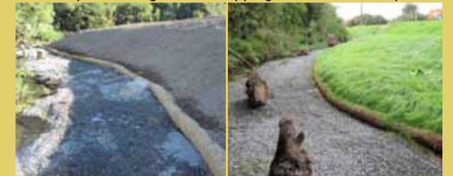
Straw Wattles were used as a major component of the Lucas Creek stream bank restoration. Our 12" Wattles were installed to protect the stream from potential sediment movement and retain topsoil on the upper slopes of the banks until vegetation was fully established. With all components of the Wattles breaking down over time they could be left in situ alleviating the need for further ground disturbance at a later time.
