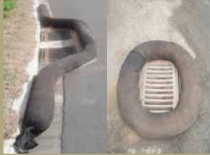
A series of Erosion Control Socks to form check dams reducing water velocity and potential scouring during high rainfall periods.
